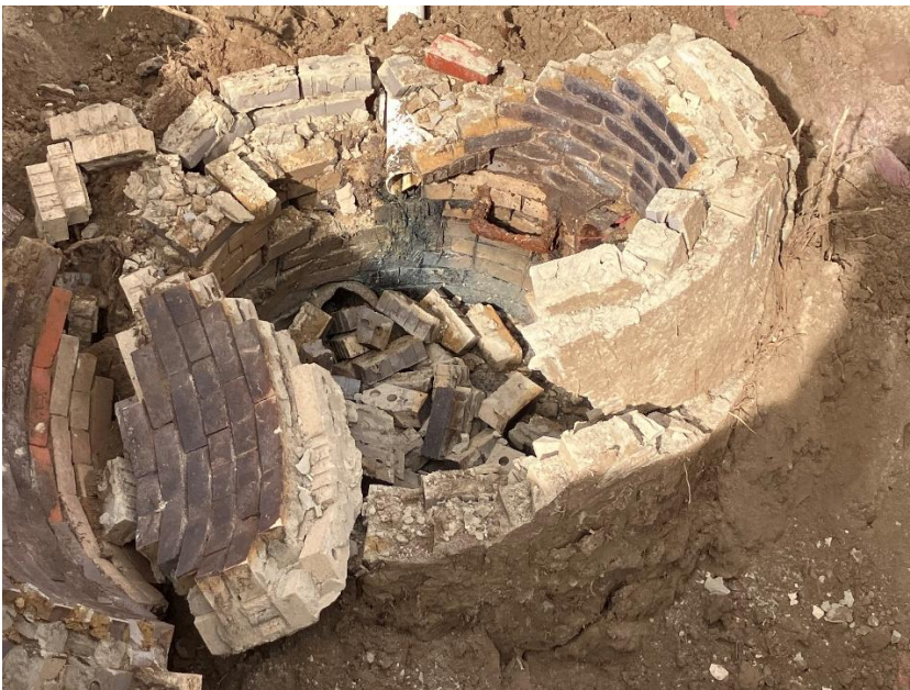
Removal of old brick manhole
