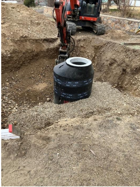
Placing Bedding
