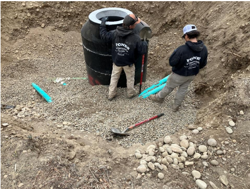
Rerouted service lines-Verified proper slope
