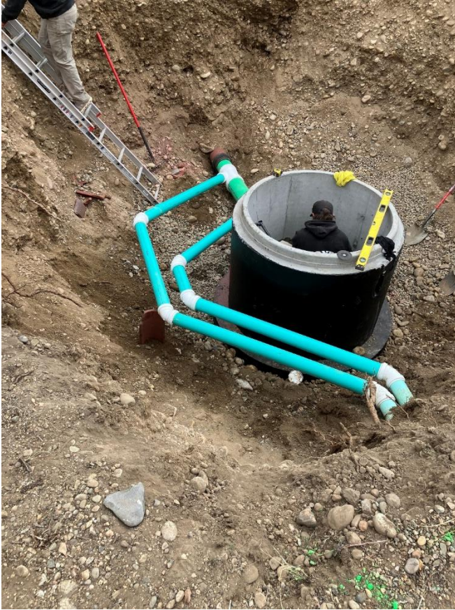
Rerouted service lines-Verified proper slope
